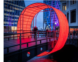
B The Clew by Ottotto Cubitt Bridge
